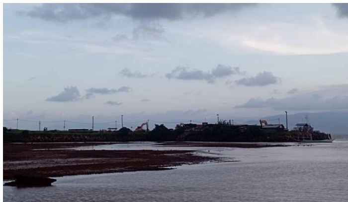
Figure 3. Condition of Mosolo Raya Due to Mining Activities 41
